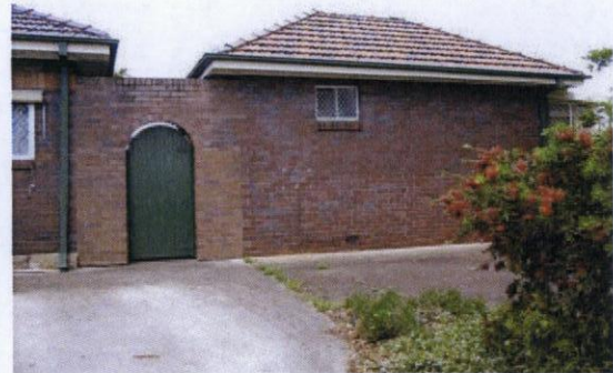
Figure 33: Enclosed courtyard and rear addition.
