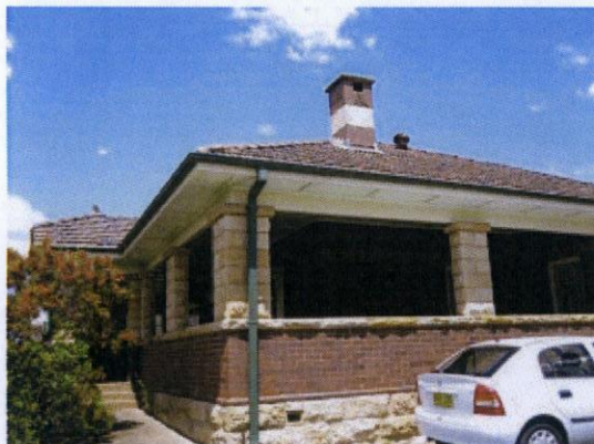
Figure 28: North elevation showing verandah stairs (to the left of frame) and chimney.
