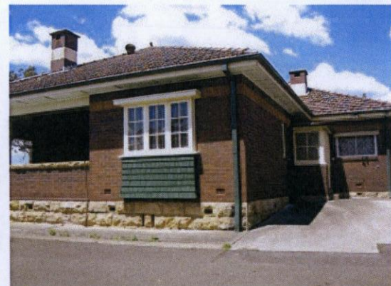
Figure 29: Detail of window at the end of the verandah on the north elevation with shingled bay.
