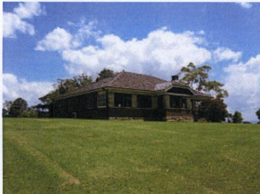
Figure 26: East (front) and south elevations of the former Farmhouse.
