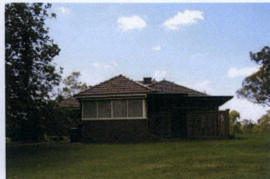
Figure 35: West elevation of the former Farmhouse.
