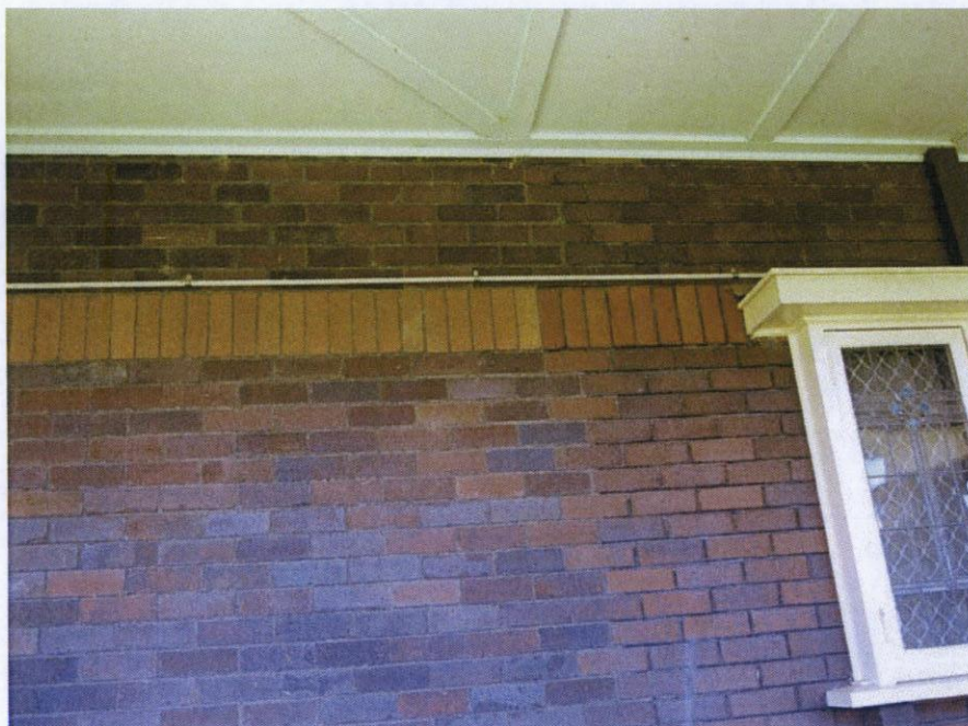
Figure 43: Detail of the join in the brickwork and soldier header row to the south end of the verandah showing location of infill.
