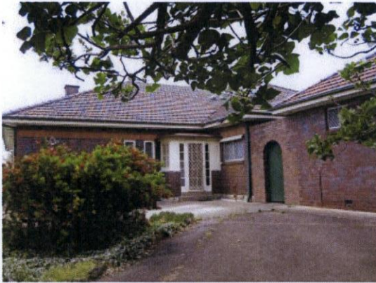
Figure 30: View to rear entry and enclosed courtyard linking the rear addition to the main house.
