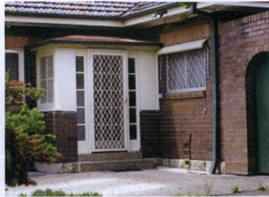
Figure 31: Detail of rear entry enclosed portico.
