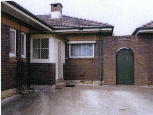
Figure 32: North elevation of rear entry and enclosed courtyard linking the rear addition to the main house.
